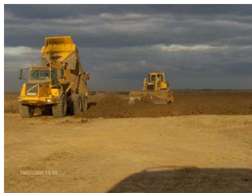
Photograph 2: Sea wall under construction
