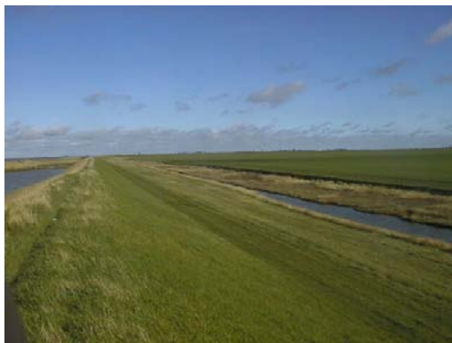
Photograph 12: Borrow dyke in Area B before realignment
