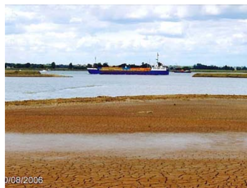
Photograph 4: One of six completed breaches viewed from the new sea wall
