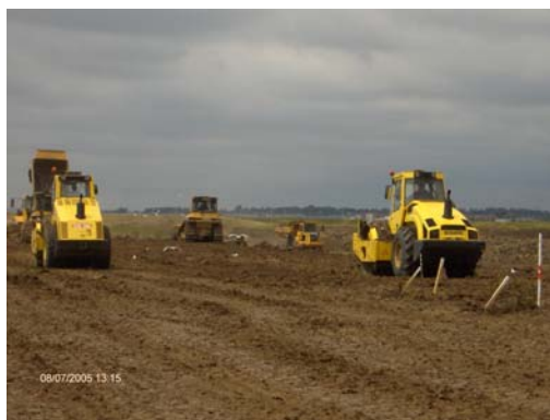
Photograph 1: Sea wall under construction
