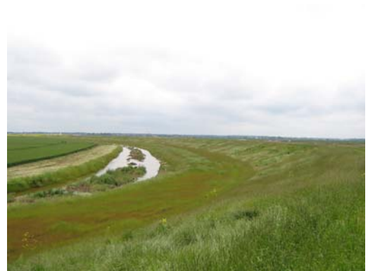
Photograph 13: Borrow dyke behind Wall B after realignment
