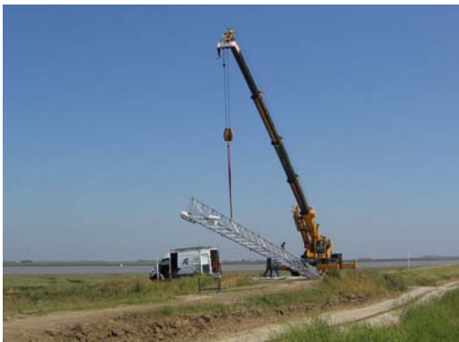
Photograph 16: New web camera tower being erected
